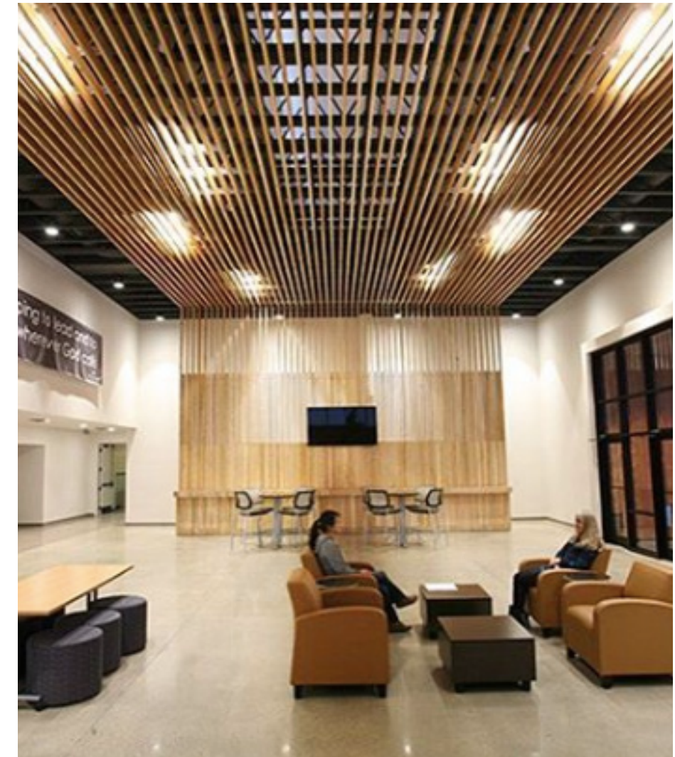
Stillwater High School required a lobby, community center, and senior thesis presentation area adjacent to the gymnasium and soccer fields. With a limited budget, 100 Fold Studio designed a 2x6 wood stud enclosure providing stadium seating, cafe seating, and a noise-reducing screen.
