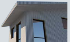
Deep eaves aid in passive solar cooling and help keep rain away from the walls
