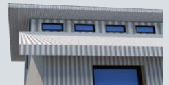
Clerestory windows bring daylight into the living area and allow for passive cooling
