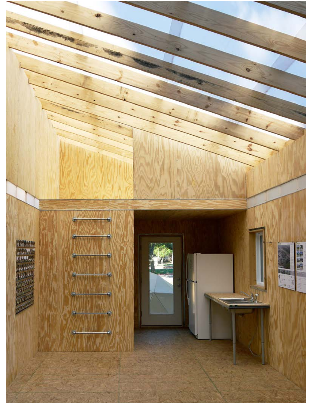
The interior of an unexpanded CORE unit makes use of panelized assemblies to ease construction means and simplify disassembly. Additionally, plumbing for the restroom (to left of the door) and the kitchen is congregated at the entry to reduce initial and long-term construction costs.
